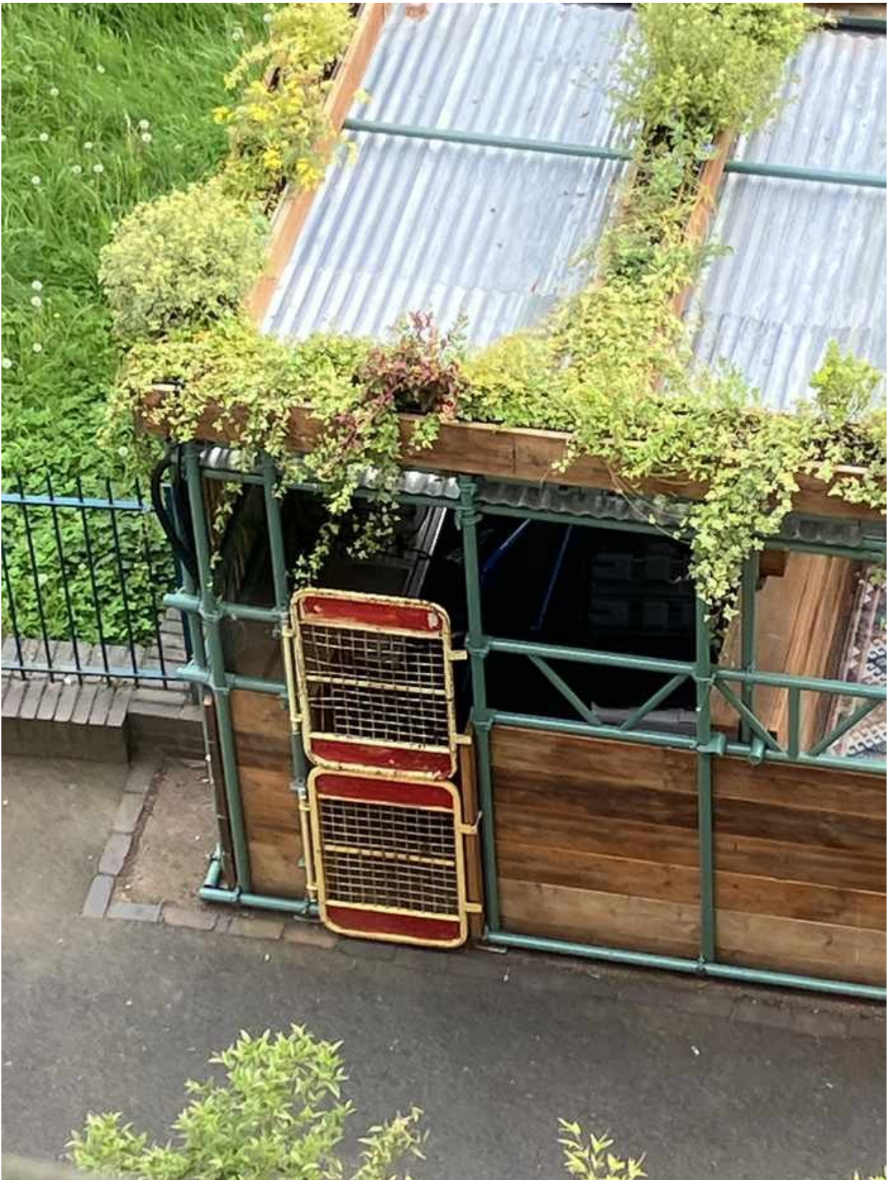
Photograph 2: Close-up structural detail showing the corrugated metal roof section, solid timber planking, and green metal scaffolding poles — all acoustically reflective materials.
