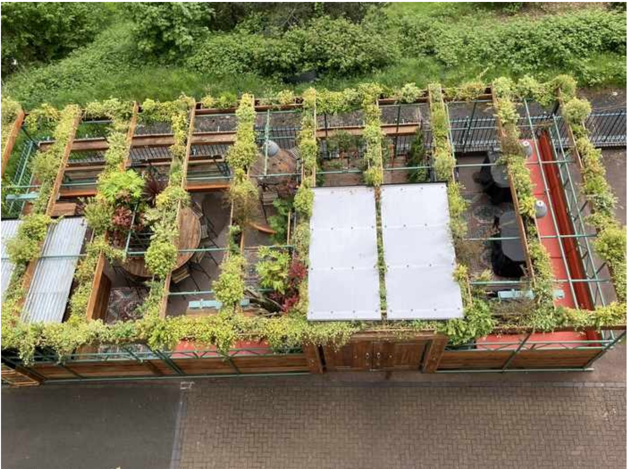
Photograph 1: Overhead view from The Court. Shows the open pergola roof structure, green metal scaffolding frame, timber wall sections, polycarbonate panels, and the direct line of sight from the residential windows above to the seating area below.
